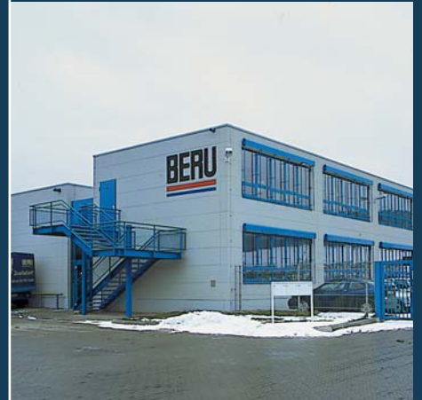
The Beru plant at Neuhaus-Schierschnitz: the industrial ceramic production factory belongs to Beru since 1991 and has been continually expanding ever since then.
